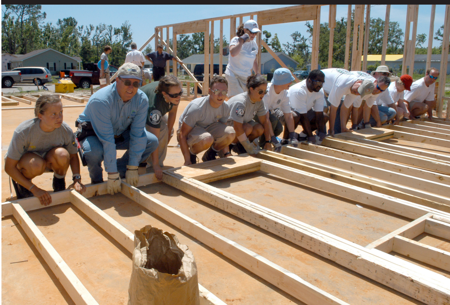
Habitat for Humanity, AmeriCorps NCC and Starbucks corporate volunteers build a bunkhouse for volunteers assisting in recovery efforts, Gulfport, Mississippi, 2006. Photo courtesy of George Armstrong/FEMA
