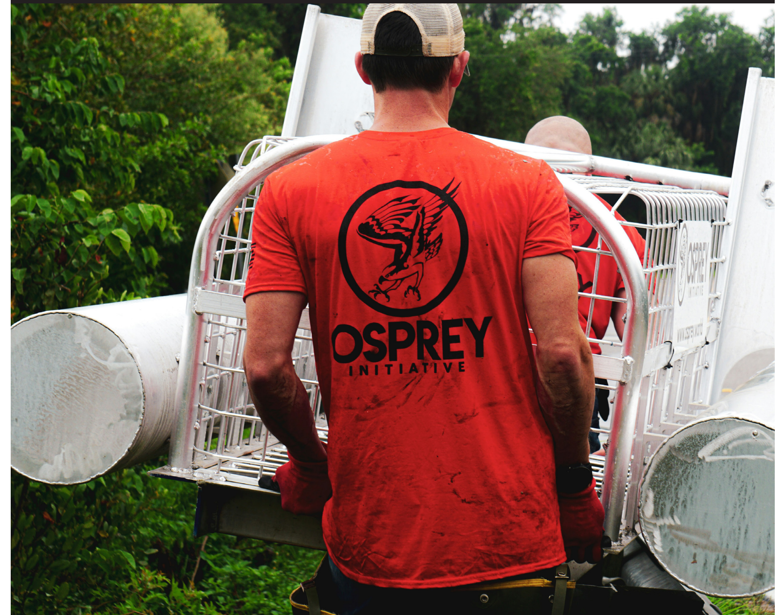
Installing a trash guard to reduce marine debris, in Ellenton, FL. with the Tampa Bay Estuary Program.
