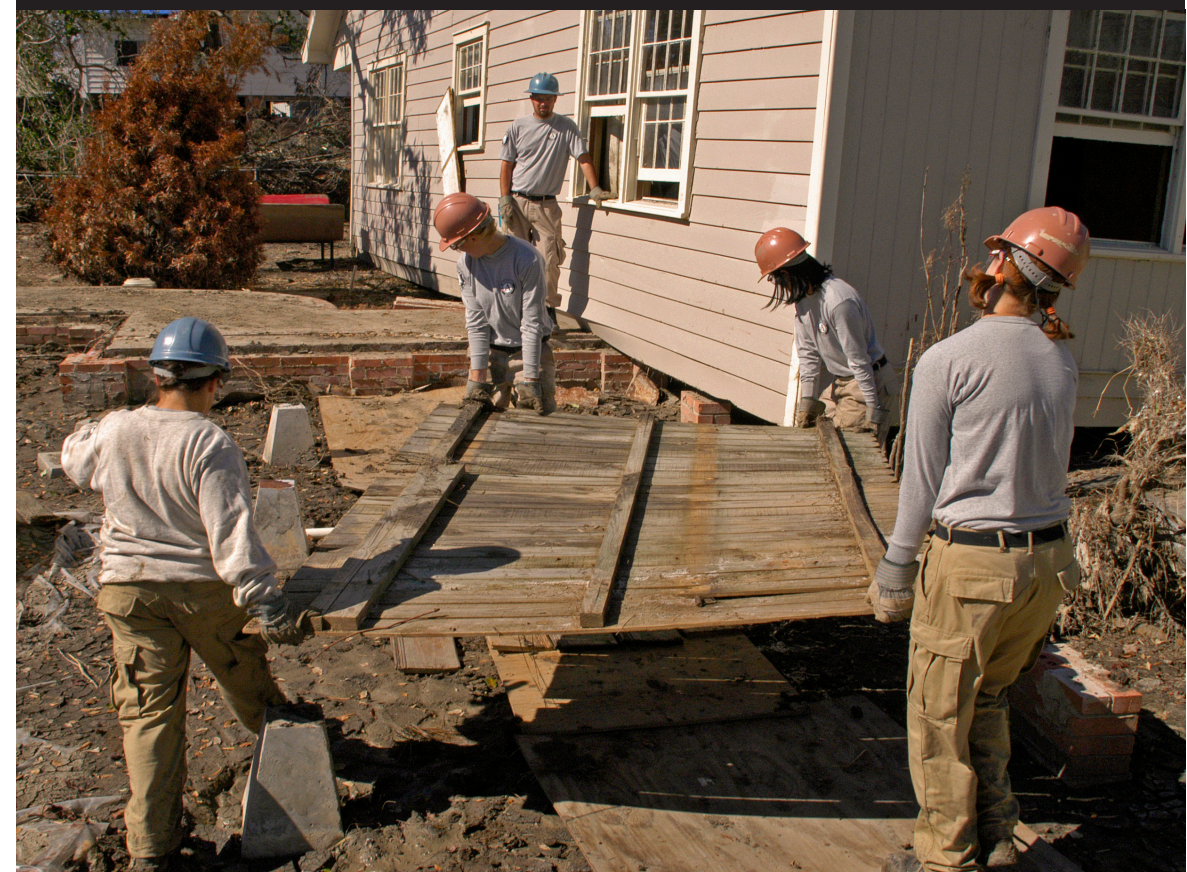
Volunteers assist with debris cleanup in Cameron, LA following Hurricane Rita
