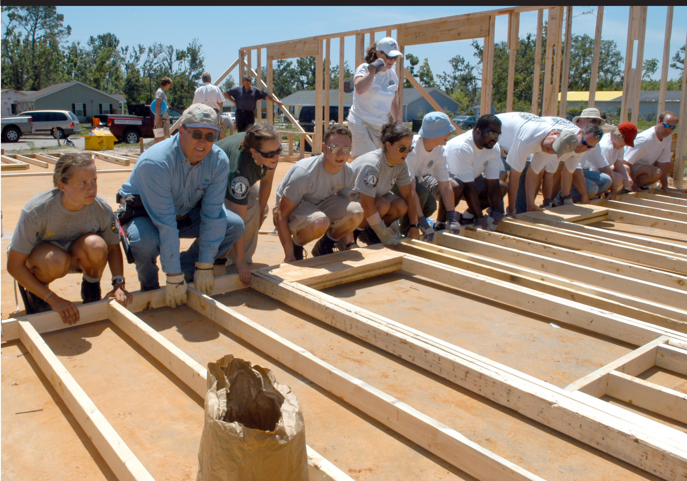
Habitat for Humanity, AmeriCorps NCC and Starbucks corporate volunteers build a bunkhouse for volunteers assisting in recovery efforts, Gulfport, Mississippi, 2006. Photo courtesy of George Armstrong/FEMA
