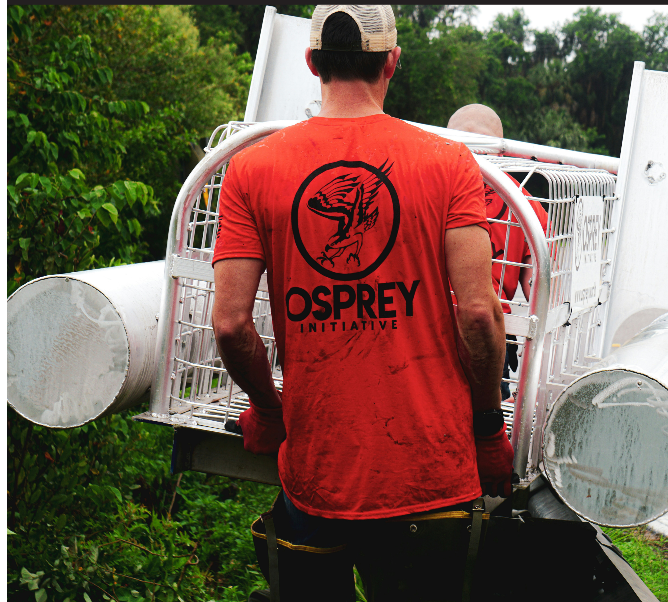
Installing a trash guard to reduce marine debris, in Ellenton, FL. with the Tampa Bay Estuary Program.
