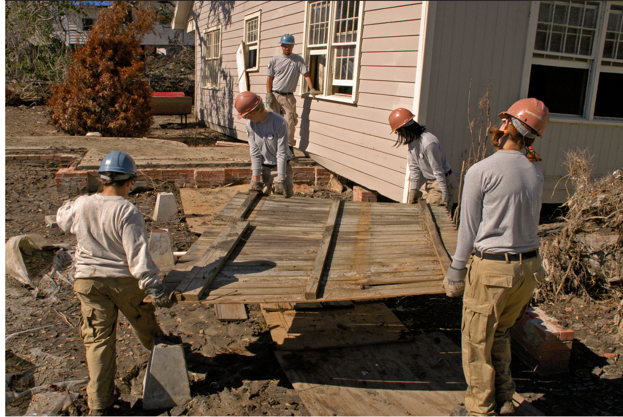
Volunteers assist with debris cleanup in Cameron, LA following Hurricane Rita
